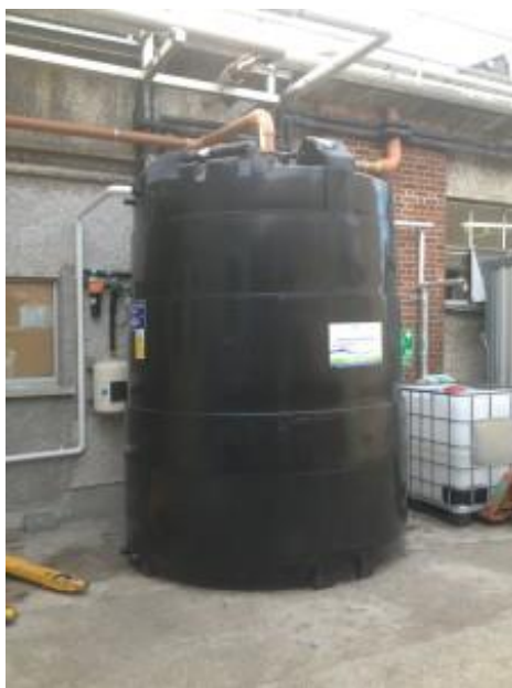
Near finished install
